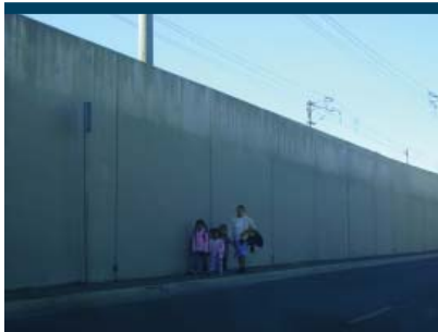
Florence Blue Line station
