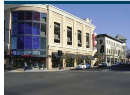
Buildings in a shared parking district
